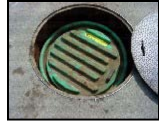
Circular steel sump lid pulled back to show the inner lid covering the turbine sump
